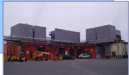
Curtain Enclosures and Barrier Walls
