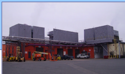
Curtain Enclosures and Barrier Walls
