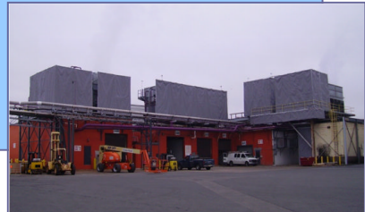
Curtain Enclosures and Barrier Walls
