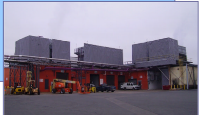
Curtain Enclosures and Barrier Walls
