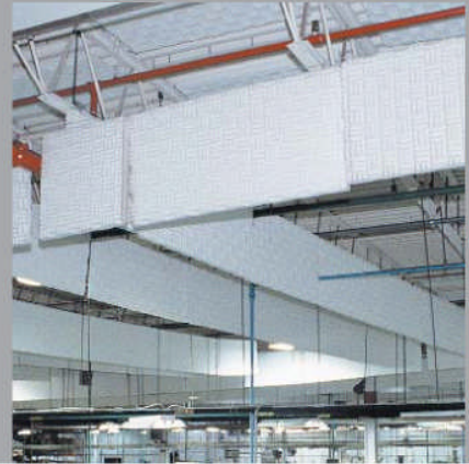
Wall-to-wall cable mount
